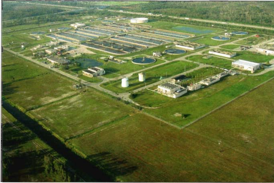
Figure 5. A reclaimed water plant producing 10 mgd for wellfield recharge and environmental restoration in South Florida
